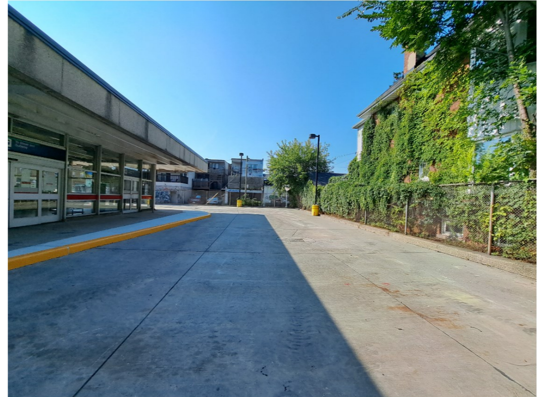
Photo: A section of the finished bus loop
