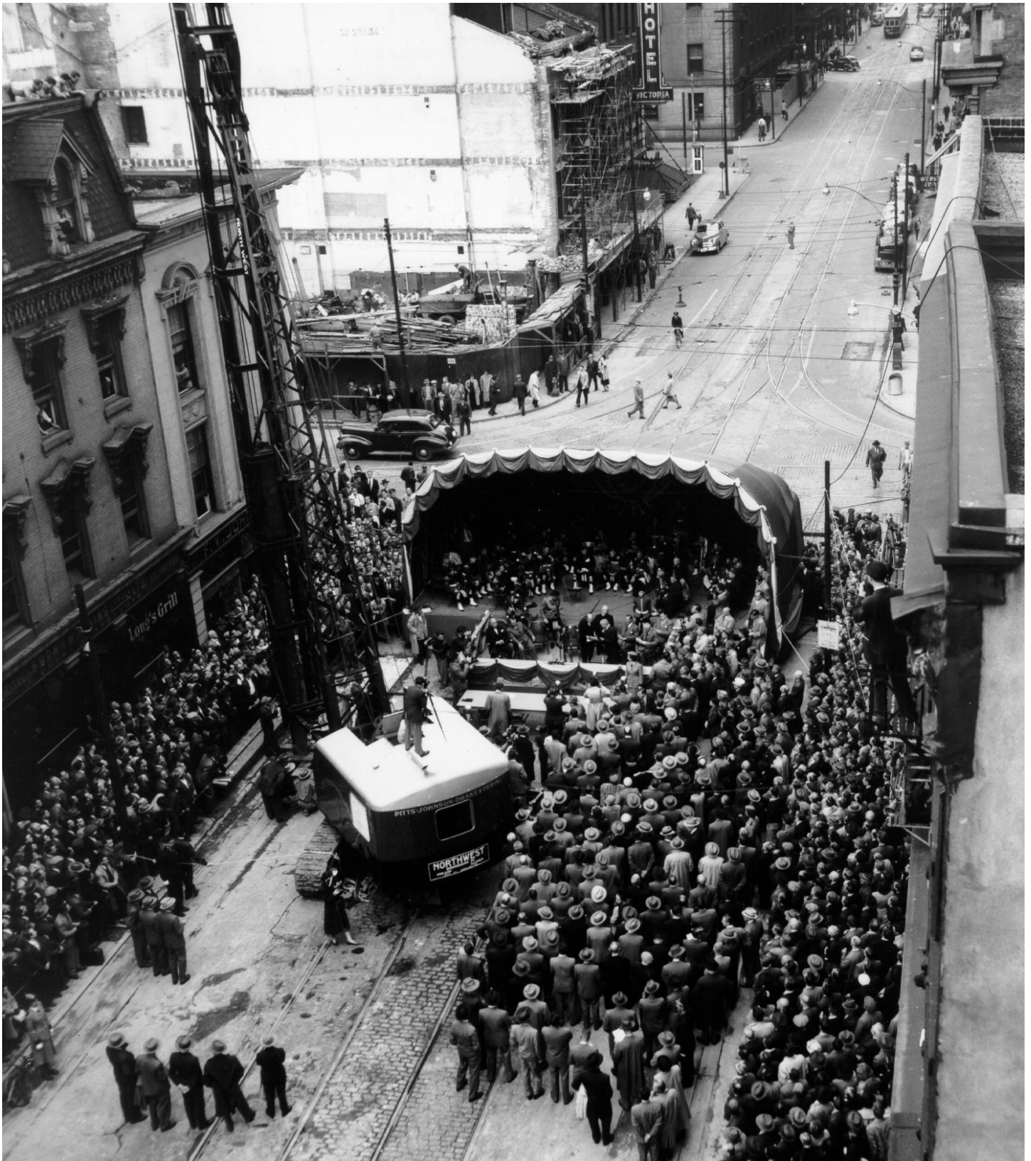
Above: On September 8, 1949: Construction began on the Yonge project, a 4.6-mile subway running under Yonge Street from Front Street to Eglinton Avenue. Construction comprised of 3.2 miles of cut-and-cover and 1.4 miles of open cut.
