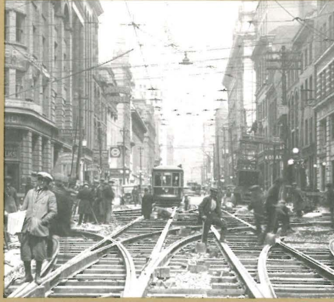
1925: Rebuilding and replacing track at Bay and Wellington Streets, part of a decade-long expansion of the network.
