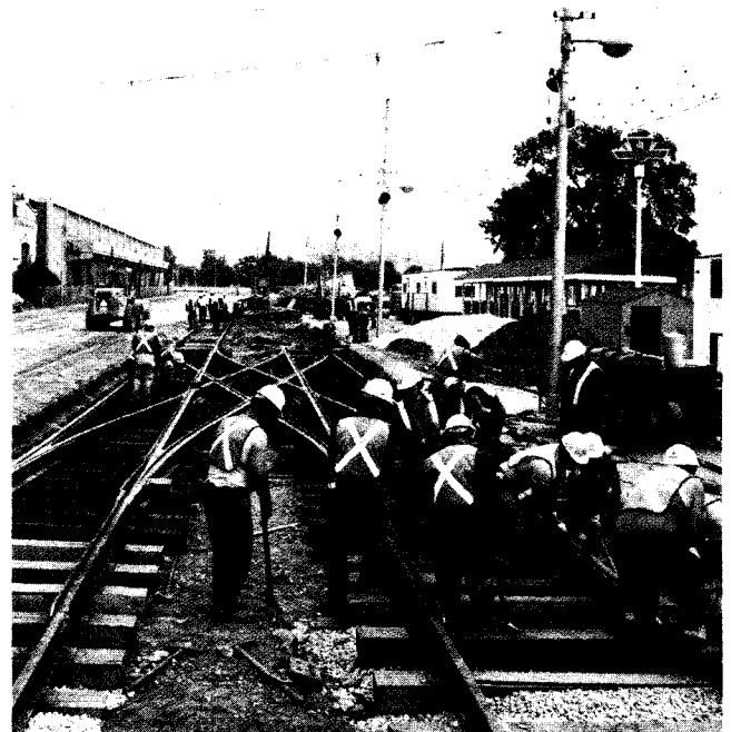
Exhibition Loop was expanded and completely rebuilt.
