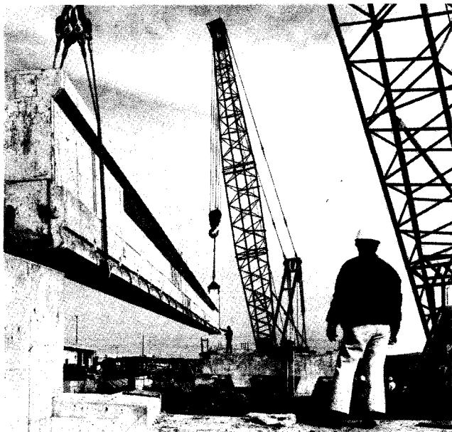
First elevated structure beam is placed on supporting piers for the Scarborough RT.
