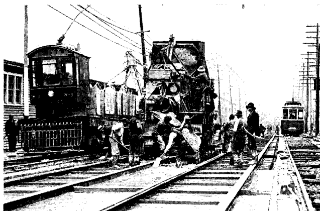
A major track rebuilding program was launched when the TTC took over in 1921. This Queen/Kingston Road view, in October 1921, shows concrete being mixed on site by the batcher and the sub-paving being poured.
