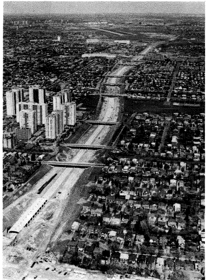
North from Eglinton West Station, the alignment of the Spadina Subway follows the median of the Allen Expressway and arterial road.
