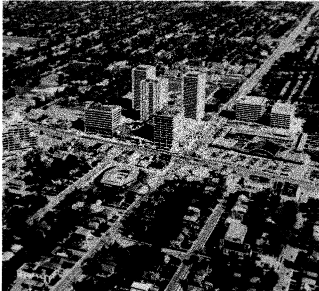
Aerial view of Yonge/Sheppard area
