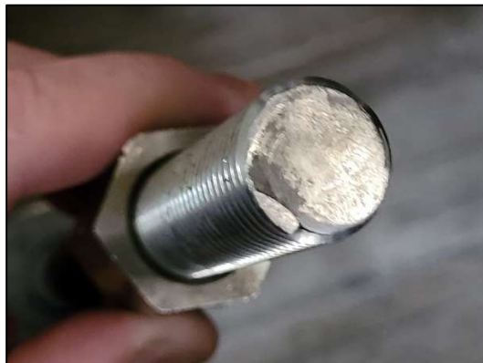
Figure 24 - Anchor Bolts #1 and #3
