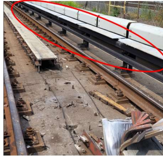
Figure 21 - 600V Contact Rail Assembly at Accident Site
