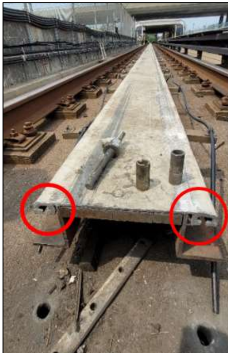
Figure 26 - Aluminum Top Cap of Reaction Rail Section A
