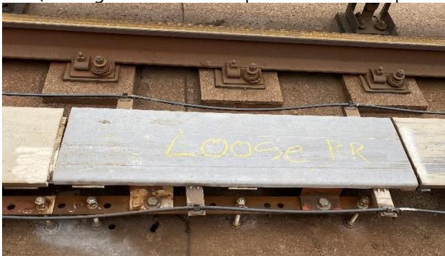
*Figure 19: Retrofit south of the derailment site, short segment with coincident joints in aluminum cap and inductor*
