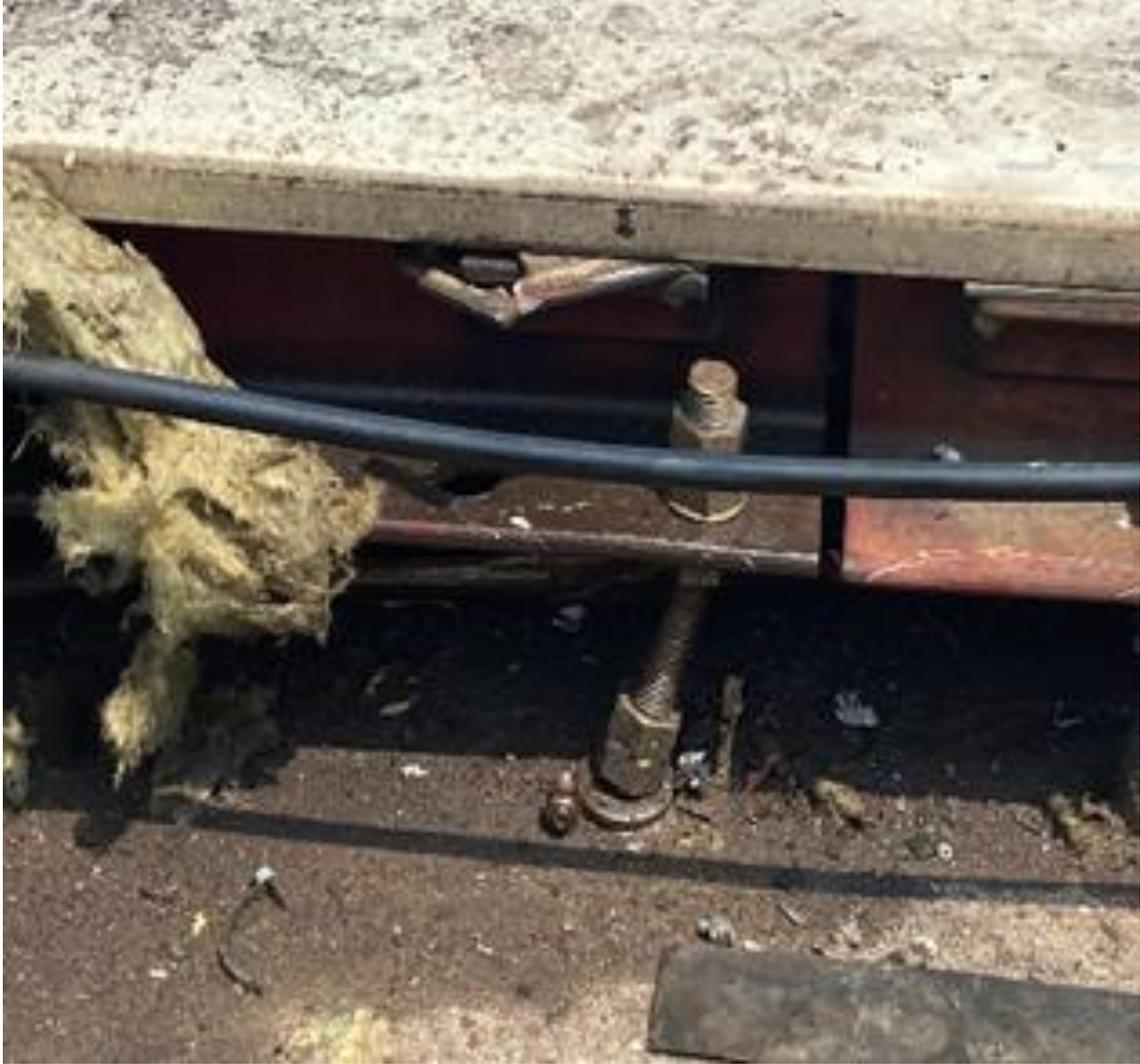
*Figure 5: Bent Anchor Bolts immediately South of Derailment Site*
