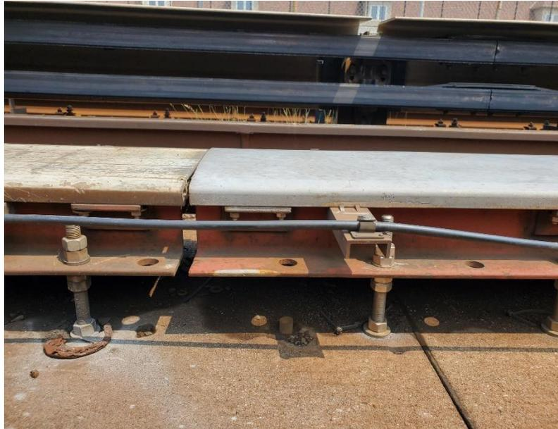
*Figure 10: Maintenance activity at similar jointed reaction rail location south of derailment site*
