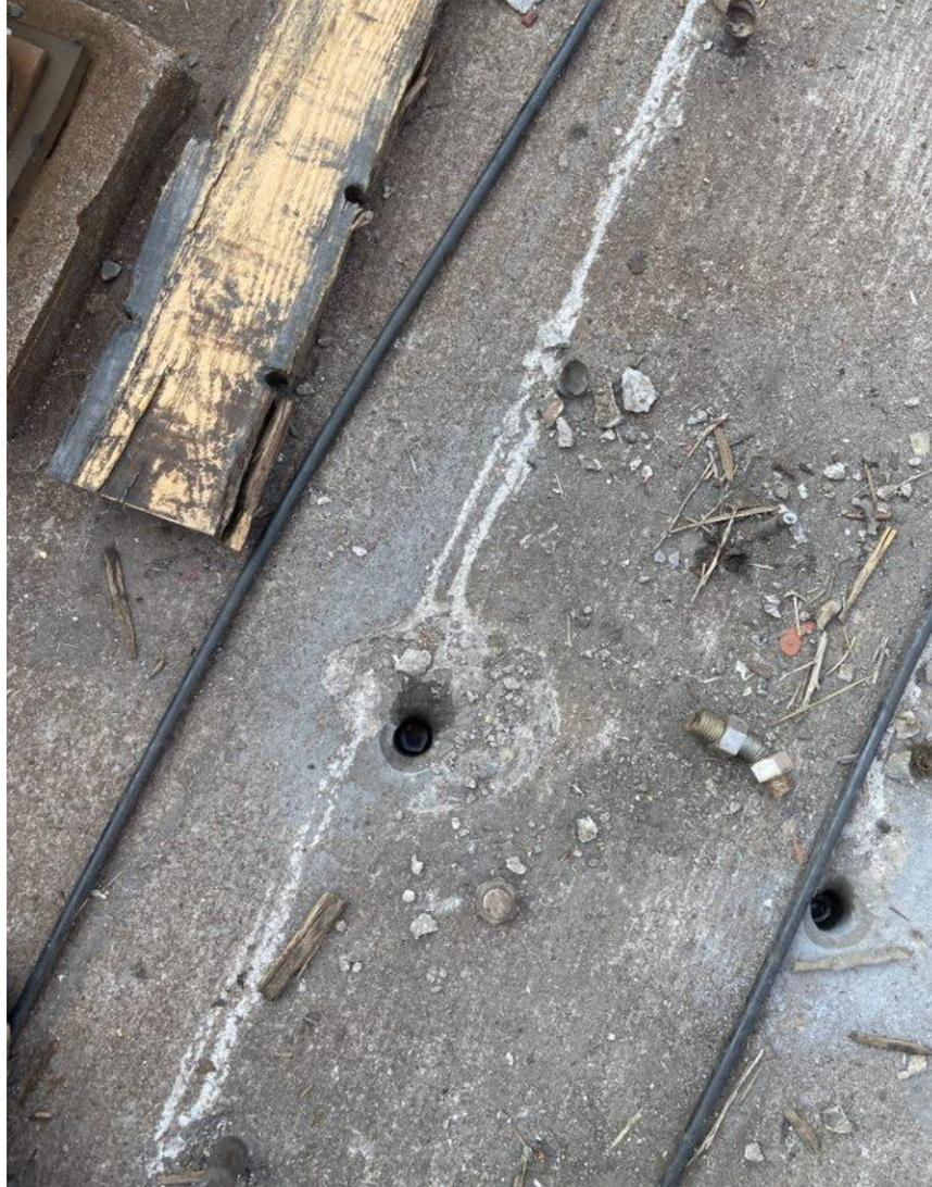
*Figure 6: Anchor Bolts pulled out of Concrete Slab*
