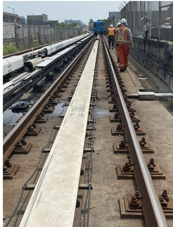
*Figure 9: Top cap abrasion on reaction rail north of derailment site*
