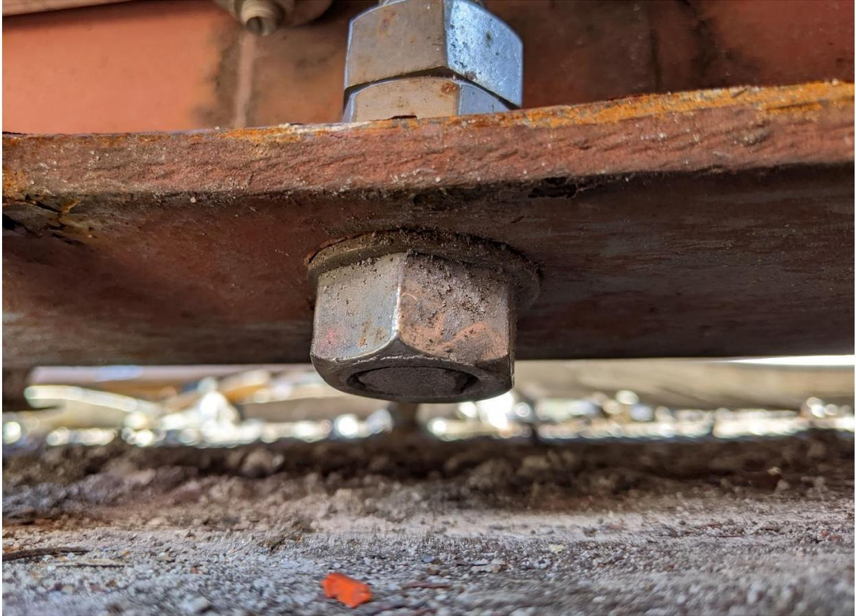
*Figure 14: Upper Portion of Anchor Bolt Attached to Reaction Rail Frame (Anchor No. 3)*
