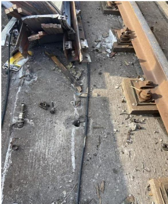
*Figure 3: Damaged Reaction Rail and Bent Anchor Bolts*
