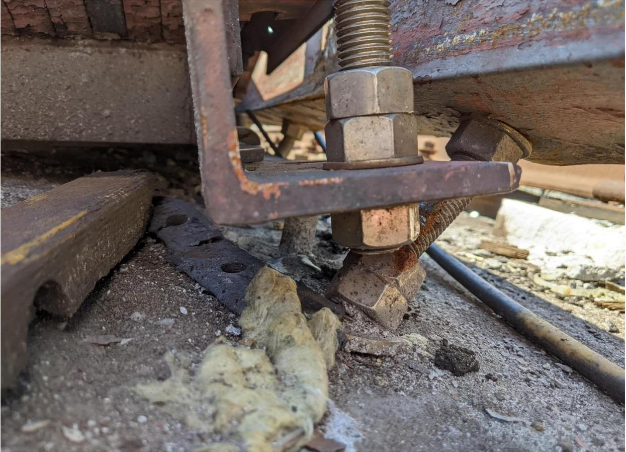
*Figure 13: Upper Portion of Anchor Bolt Attached to Reaction Rail Frame (Anchor No. 1)*
