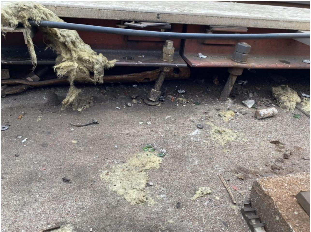
*Figure 8: Bent Anchor Bolts South End of Derailment Site*
