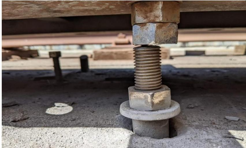
*Figure 15: Fractured anchor bolt located approximately 70m south of the derailment site*
