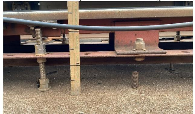
*Figure 20: HSL-GR M20 anchors at retrofit south of the derailment site*
