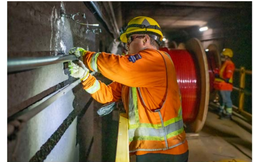
TTC crews installing cellular service cables on Line 2 (Action 2.2.4)
