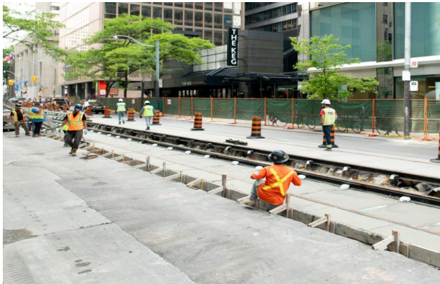
Above: Tracks being laid on York Street.
