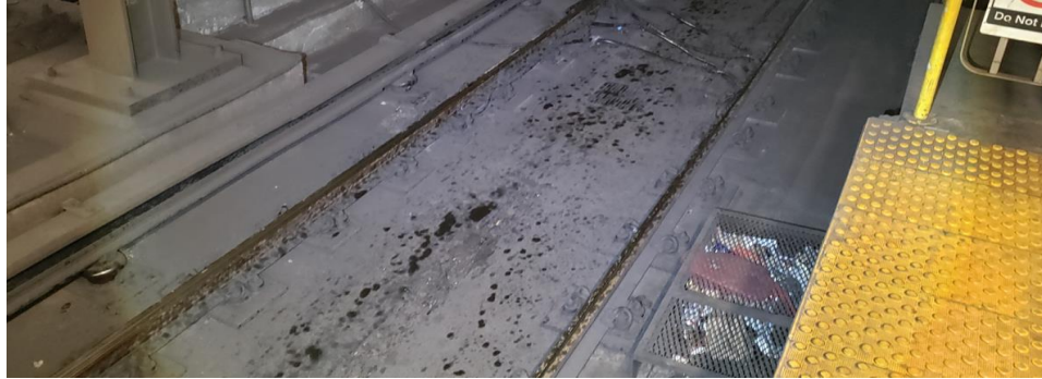
Figure 11 - Hydraulic fluid leaked on rails and track bed at Sherbourne station
