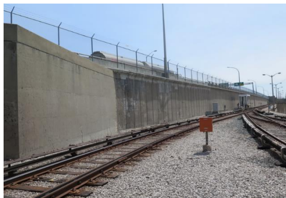
Figure 8-8: Retaining wall adjacent to Wilson Yard tracks.
