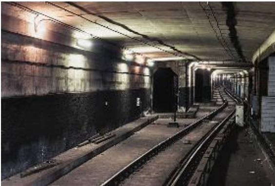
Figure 5-1: Underground subway track.
