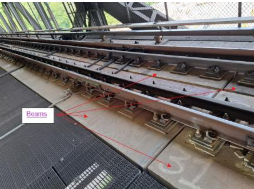
Figure 8-6: Prince Edward Viaduct beams.
