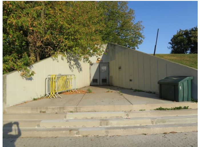
Figure 8-9: Emergency exit on Line 1 south of Eglinton West Station.
