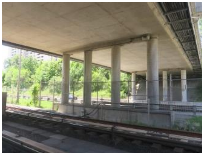
Figure 8-7: Ridelle Avenue Bridge
