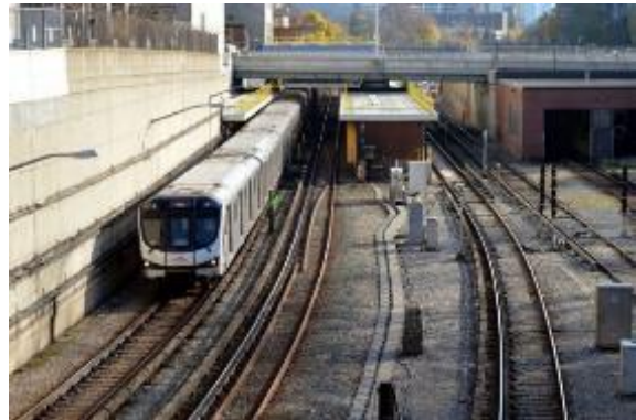
Figure 5-2: Overground subway track.
