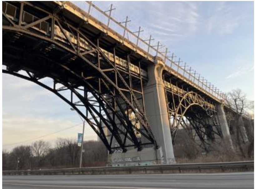
Figure 8-5: Prince Edward Viaduct.
