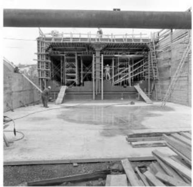
Figure 8-1: Box tunnel for Line 4.
