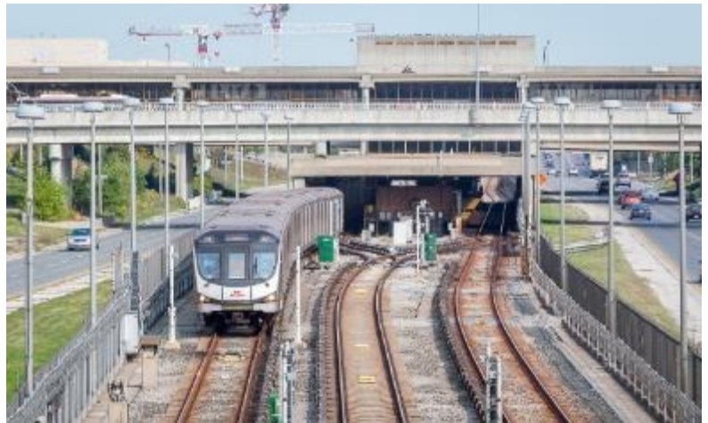
Figure 6-4: TTC Subway Station.
