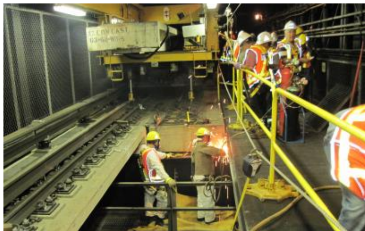
Figure 8-11: Replacing Beams on the Prince Edward Viaduct.
