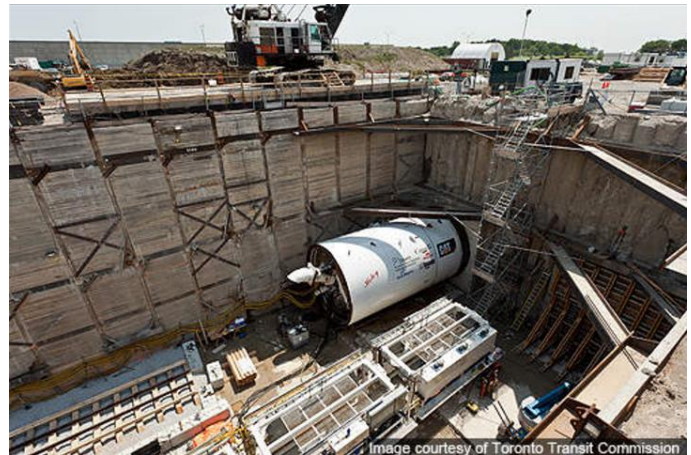
Figure 8-2: Tunnel Boring Machine for Line 1 Toronto-York Spadina Subway Extension.
