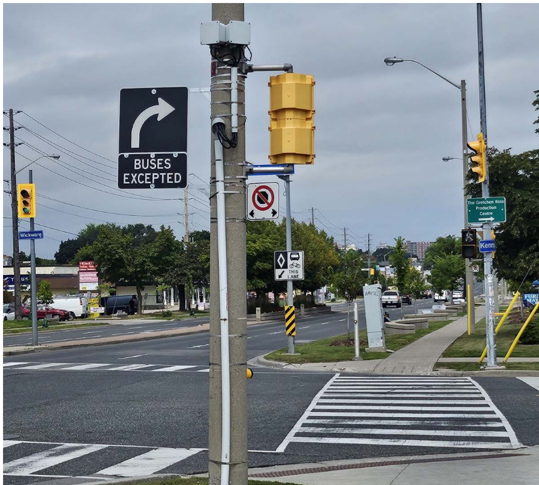
Figure 5. Kennedy Road with Signs for Bus Priority (Queue Jump and Transit Lane)
