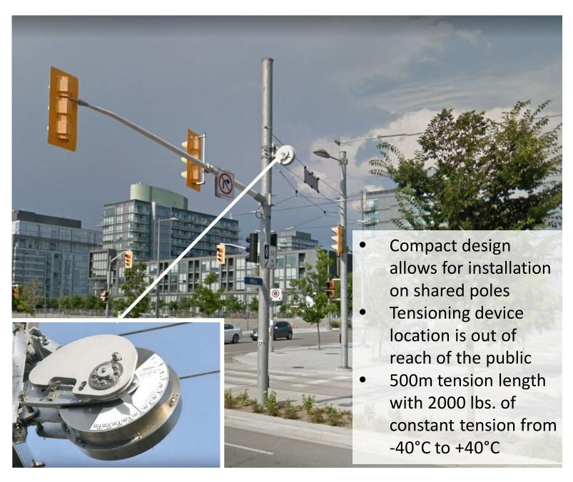
Cam/Spiral – Constant Tensioning Device
