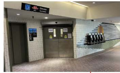
EXISTING GROUND FLOOR TTC CONCOURSE ELEVATOR
