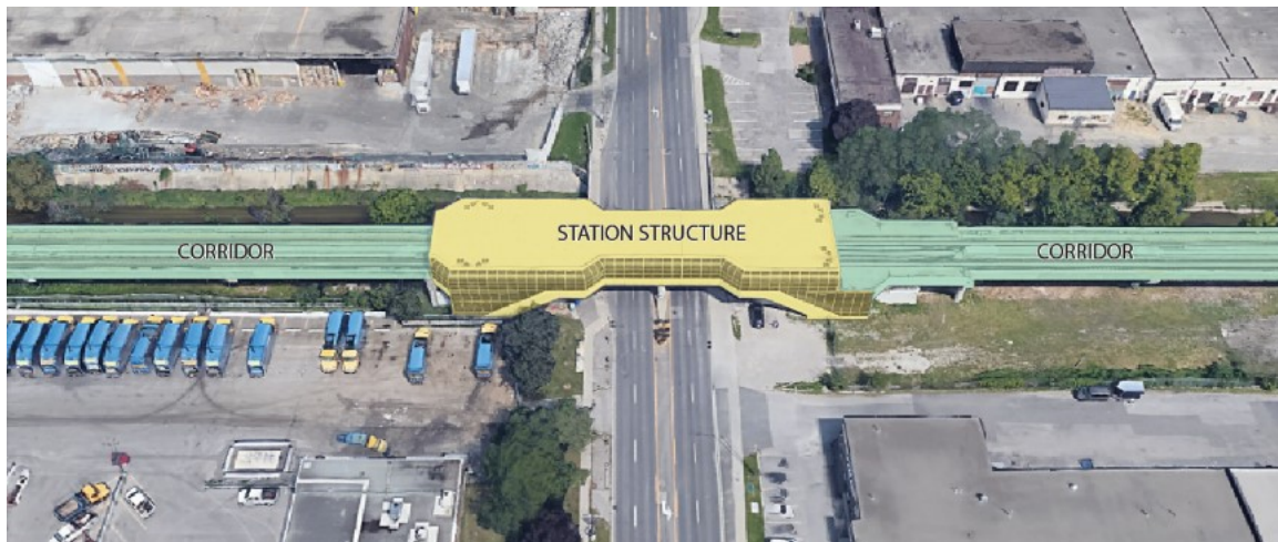
Figure 4. Image of Line 3 Infrastructure – Station Structure and Corridor Highlighted
