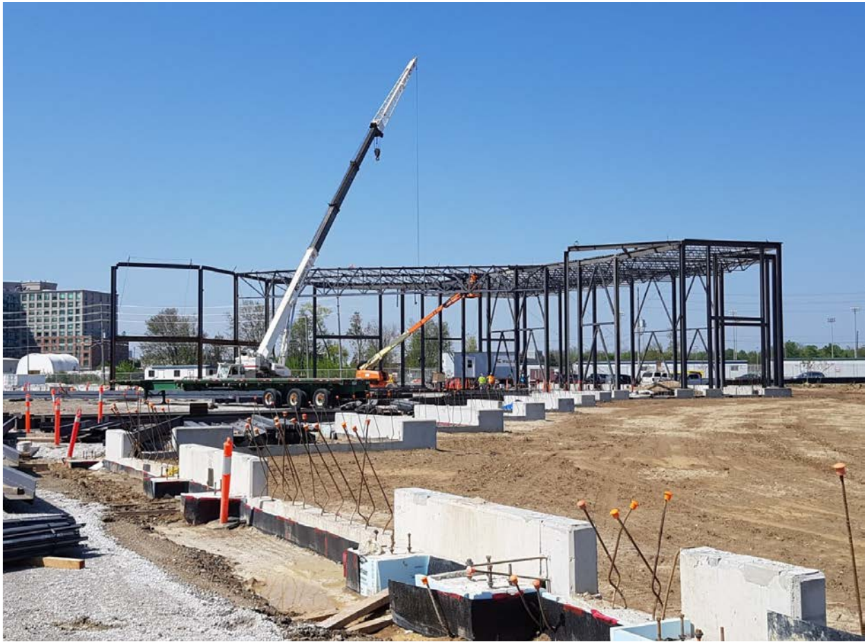
Figure 12: McNicoll Bus Garage Under Construction, May 2018
