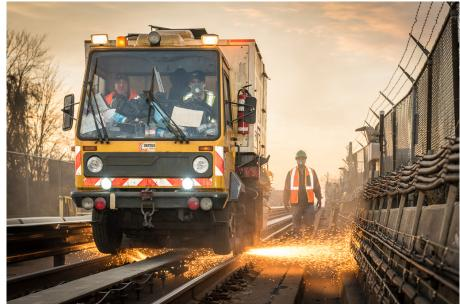
Replaced power rail, track fasteners, ties and communication cables on Scarborough Line 3
