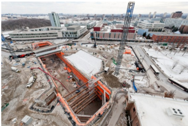
Downsview Park Station photo is a west view of concrete walls and formwork at the east end of the east building.
