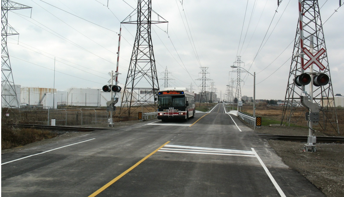
Figure 6 –Existing Busway in the Hydro Corridor
