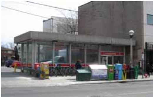
Existing East Entrance
