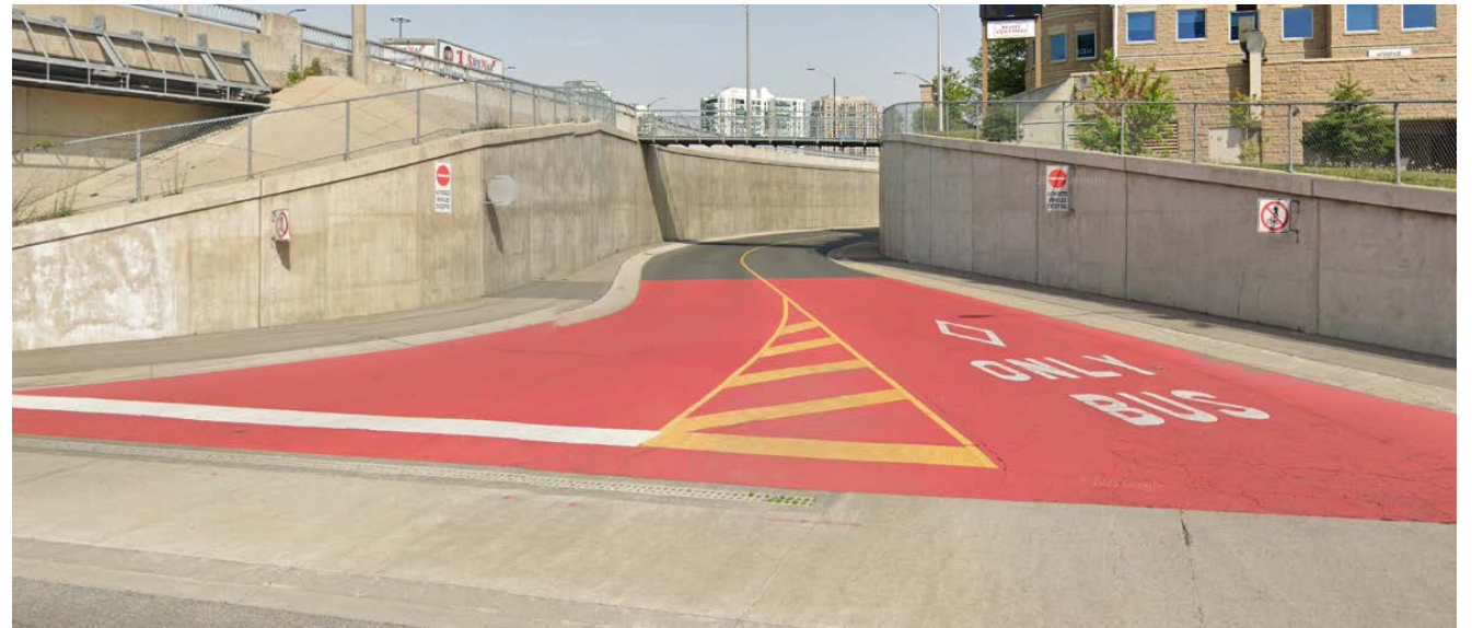
Example of treatment at Mississauga Transitway driveway
