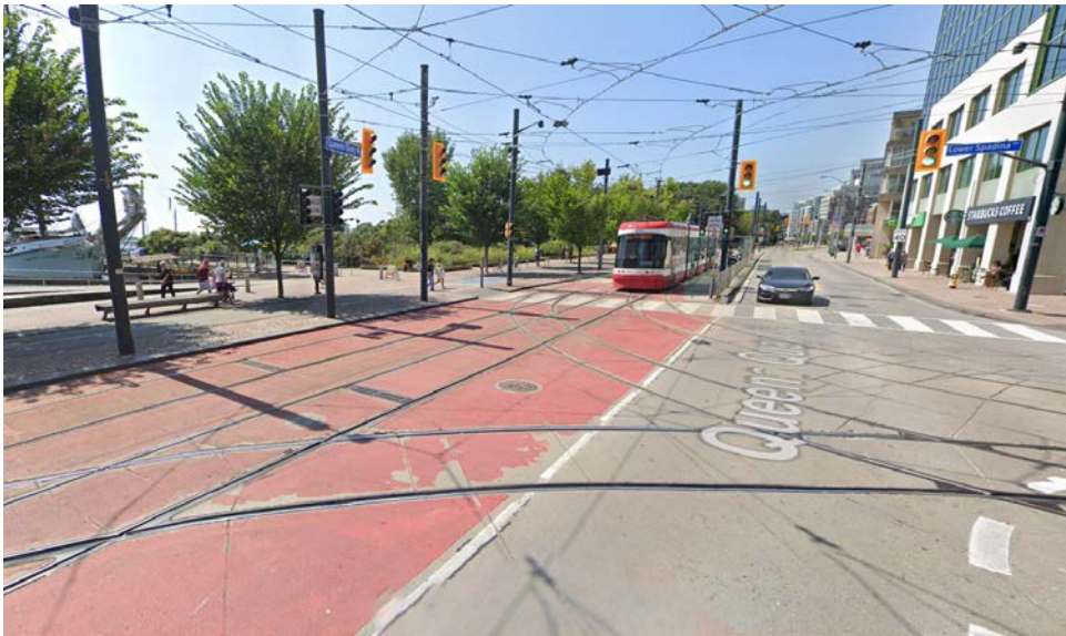
Project to expand red-paint application like at Queens Quay / Spadina (installed since 2018)
