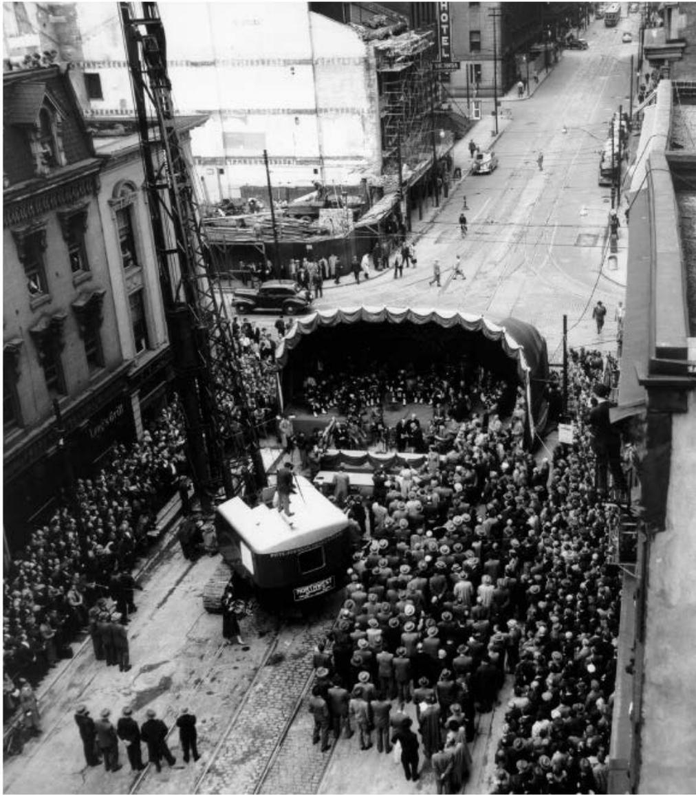
Above: On September 8, 1949: Construction began on the Yonge project, a 4.6-mile subway running under Yonge Street from Front Street to Eglinton Avenue. Construction comprised of 3.2 miles of cut-and-cover and 1.4 miles of open cut.
