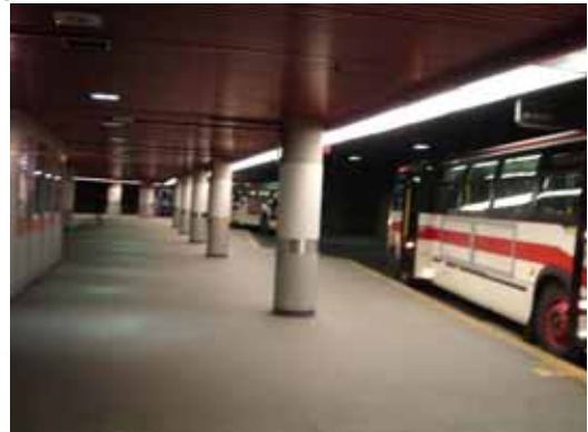
Current lighting at York Mills Station
