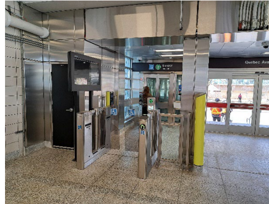
Elevators completed at High Park Station
