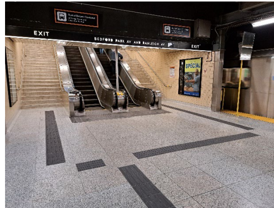
(left) Lawrence Station upgraded tactile wayfinding path
