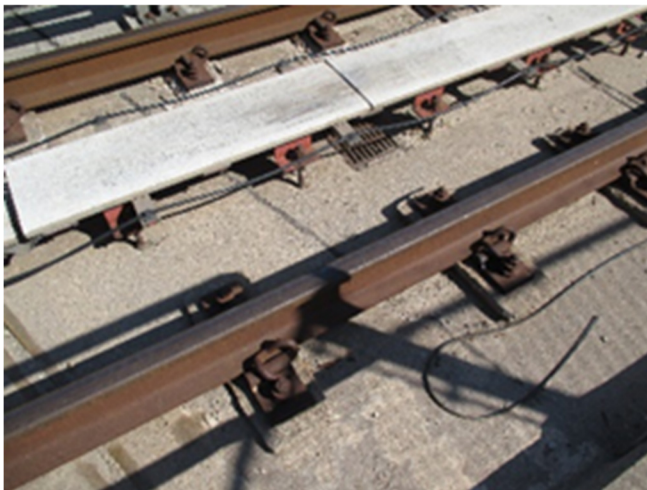
Figure 2: Wear marks on reaction rail
