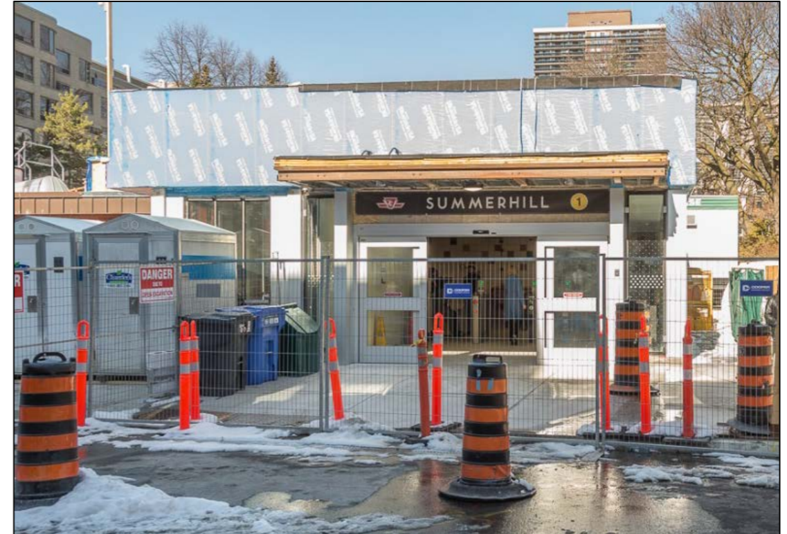
Picture- New main entrance at Summerhill Station
