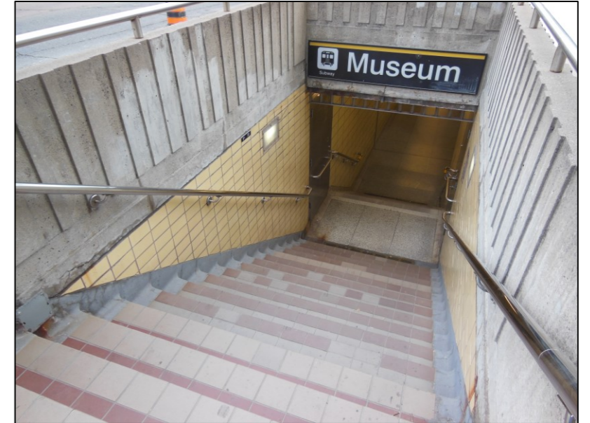
Existing stairway entrance/exit at Museum Station
