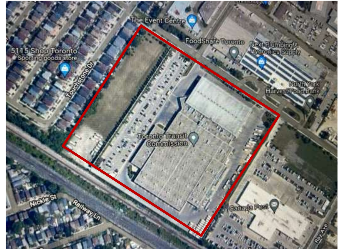
Aerial image of Mount Dennis Bus Garage
