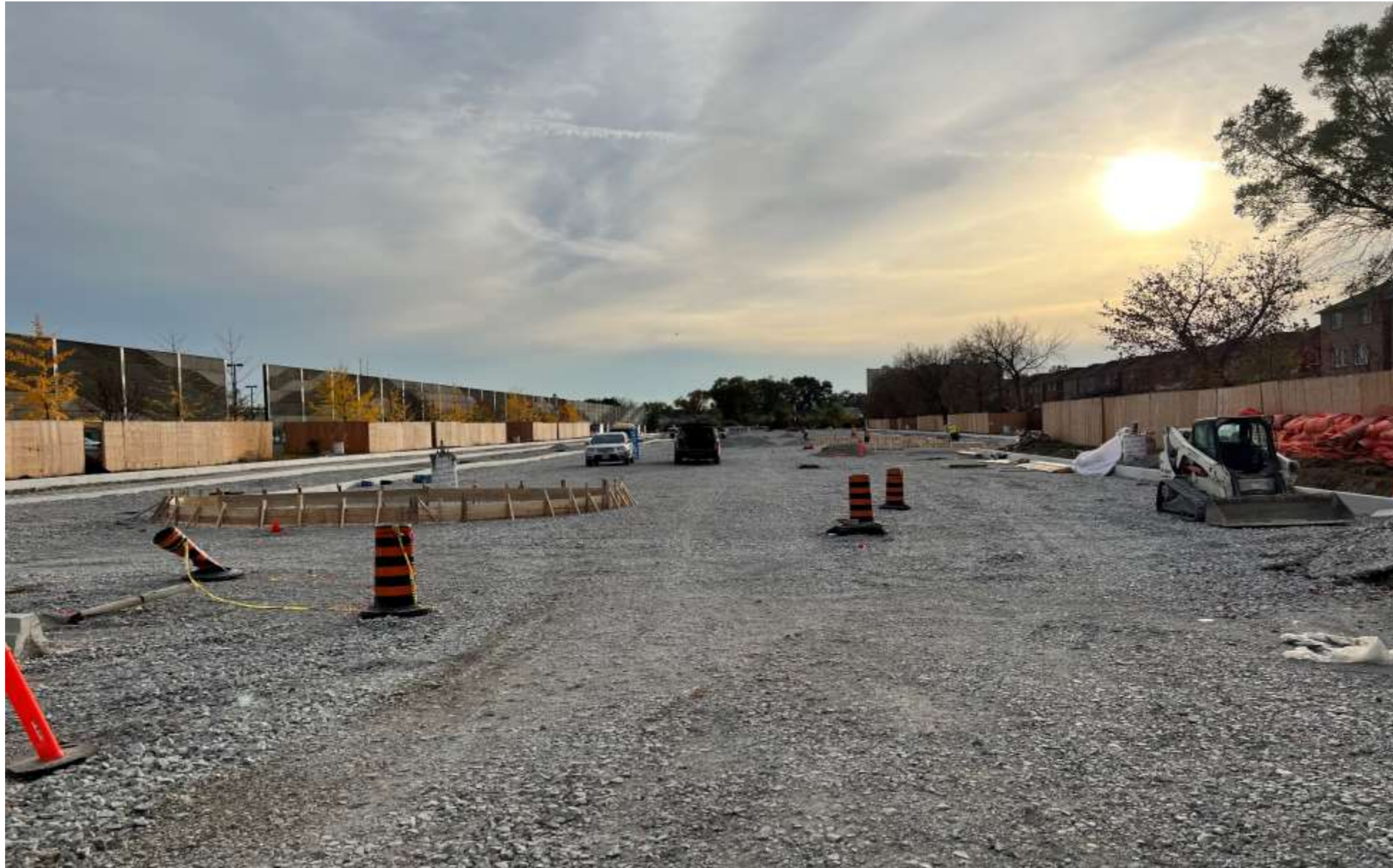
Work site as of November 3 rd , 2023, looking northwest
