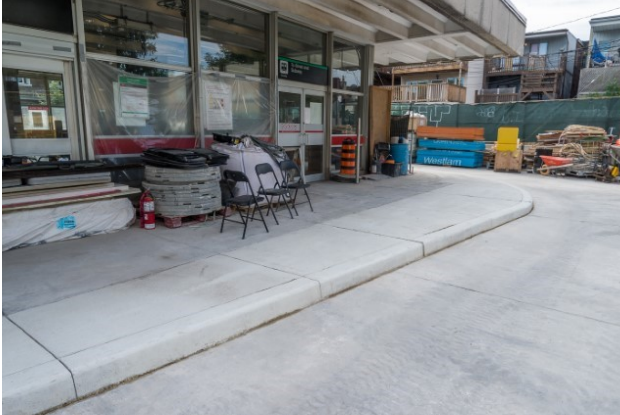
Photo: Bus loop curb completed
