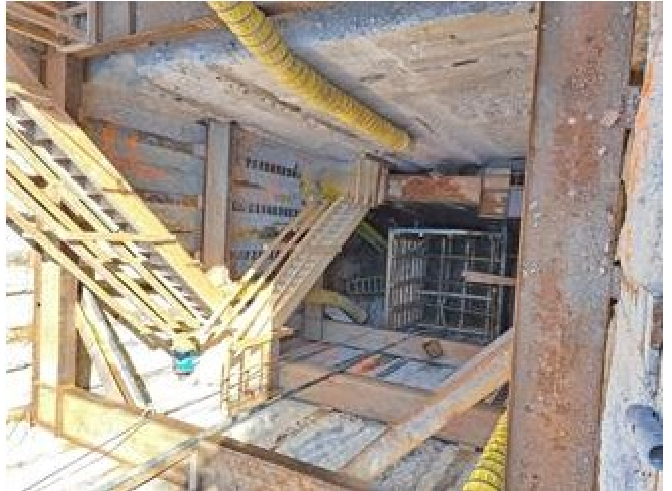
Photo: Elevator 2 excavation
