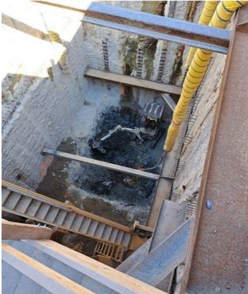
Photo: Elevator 1 excavation
