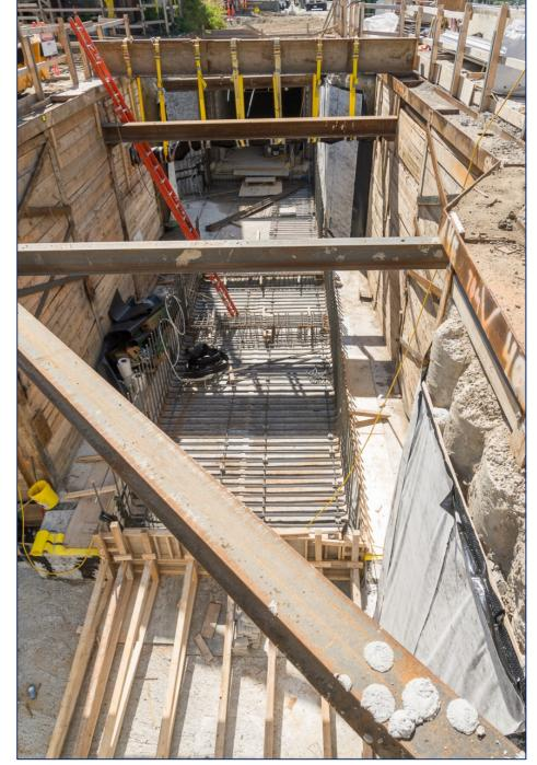
Photo - At street level facing South looking at rebar being placed between expansion joints in base slab at passageway along Dewhurst.
