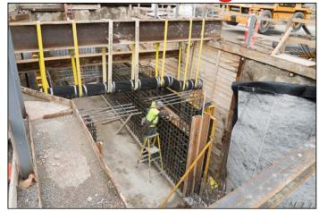
Photo – Looking NE into the Dewhurst passageway- rebar installation
