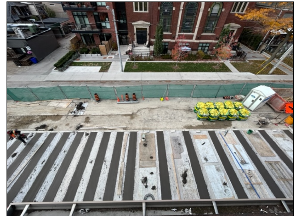
Photo – Future sidewalk on Dewhurst (passageway below)
