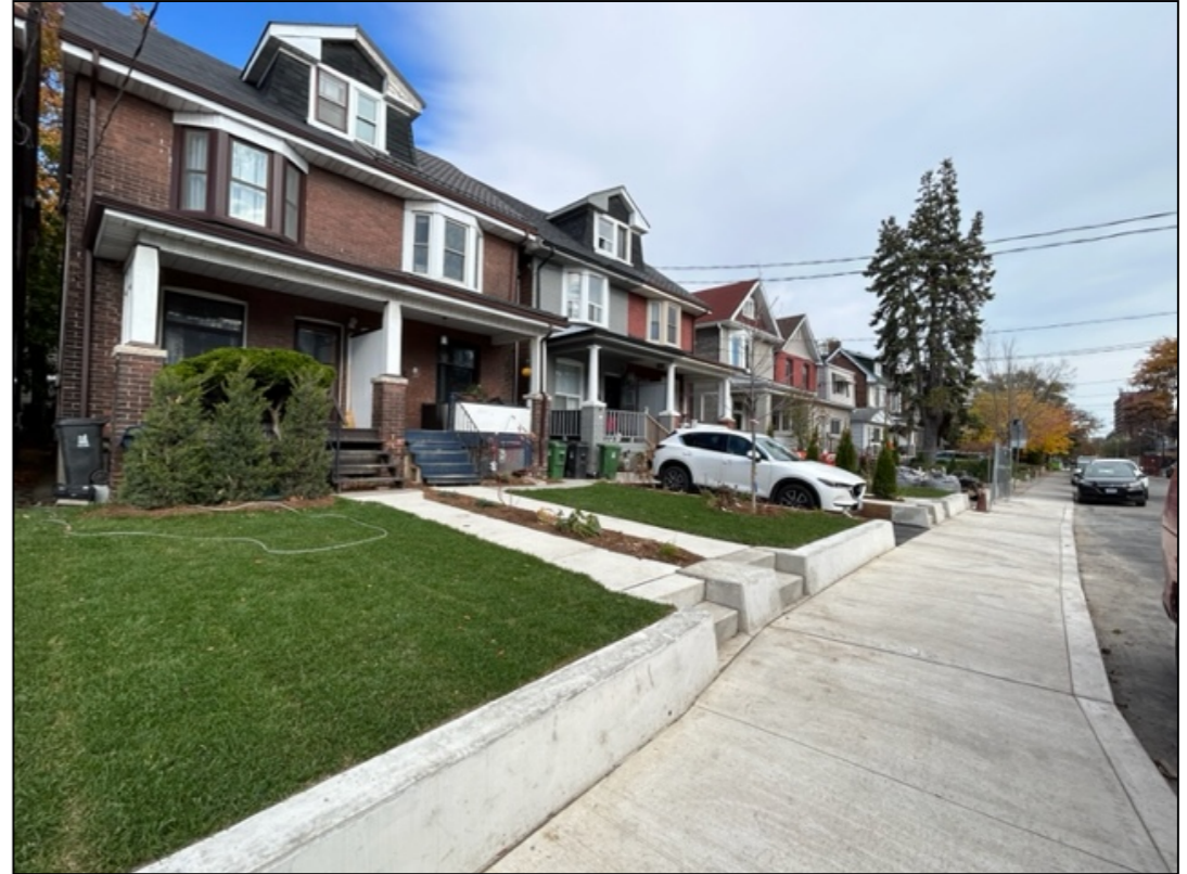
Photo – Looking east at the north side of Strathmore's restoration progress
