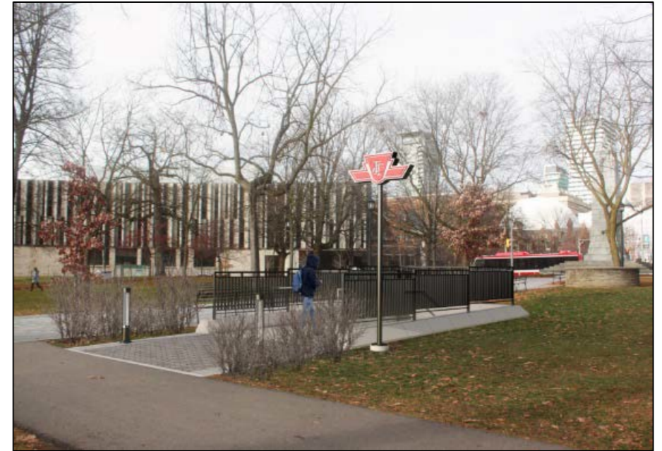
New second entrance/exit at north end of Queen's Park Circle
