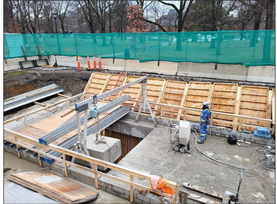
Cutting the tunnel roof at south end of Museum Station for the Second Exit/Entrance in Queen's Park Circle, looking west.
