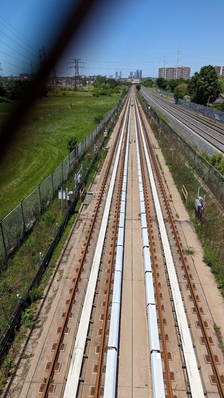
Photograph 7: Tara Road – facing North
