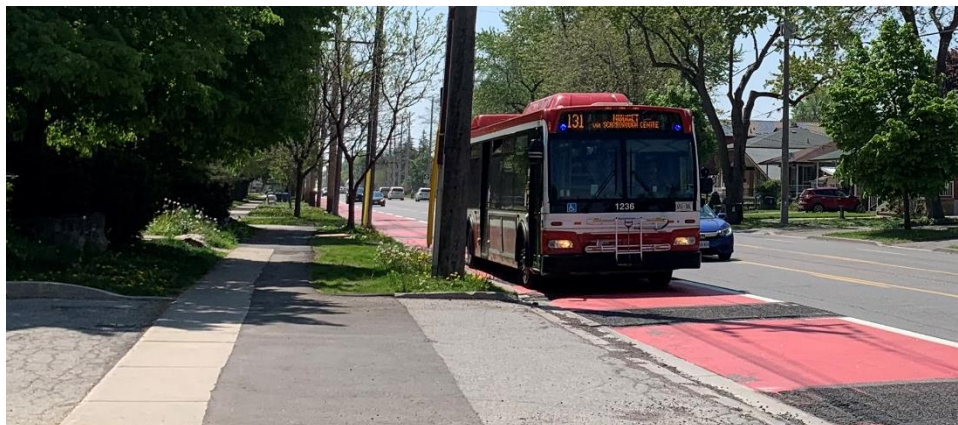
Figure 3-2: Painted Bus/Bike Lanes on Kennedy Road
