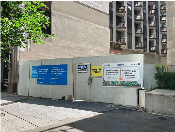
81 Bloor St E with project funding signs on construction hoarding
